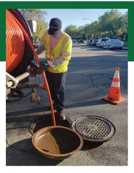
For most wastewater utilities, collection systems are 'blind spots' creating the need to routinely clean at specific sites based on a history and/or perceived risk of spills. A wastewater operator increases cleaning frequency because not only does cleaning reduce near-term risk, but more frequent visits to troubled sites gives more frequent information about the sites.
